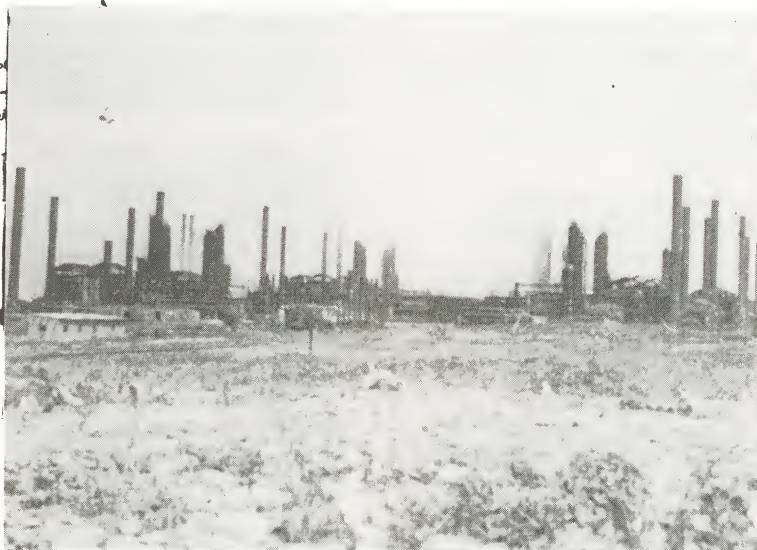
The first barrel of crude passed through Lago topping stills in 1929.
